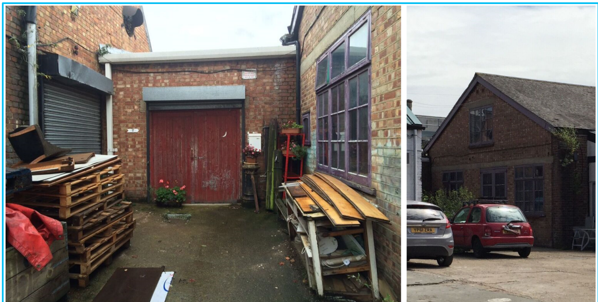
Figure 10 Existing Live/work premises
